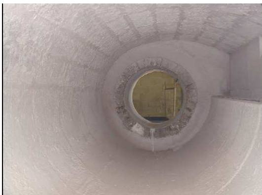
Boiler - After application of Furnascote
