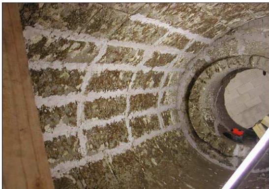
Boiler—Before application of Furnascote
